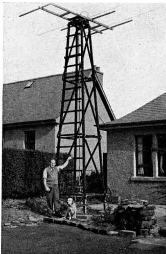
The completed 28 Mc/s. rotary beam with its owner.
